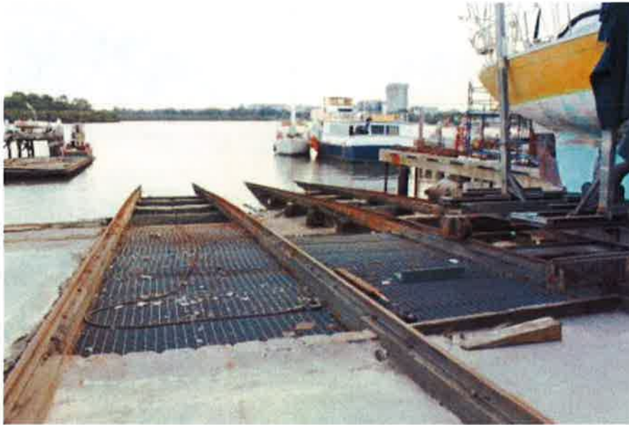
Figure 5 – The existing slipway
