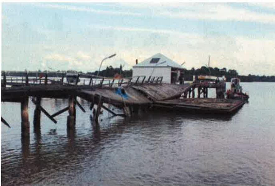
Figure 6 – Structures on the Site are in disrepair and pose safety risks
