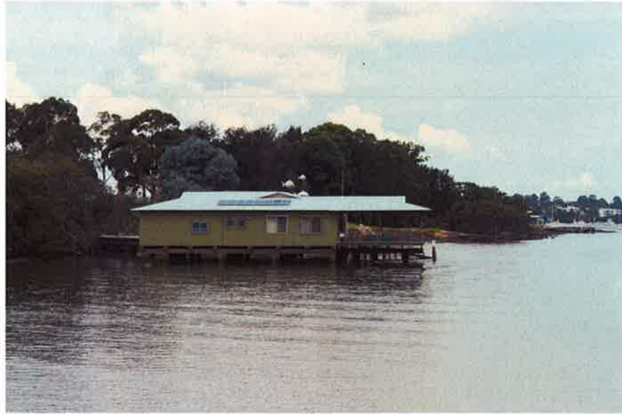
Figure 16 – Kissing Point Wharf
